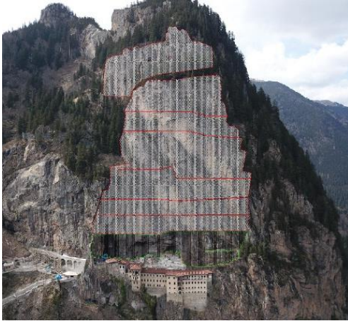
Slope area steel wire application ©MoCT
