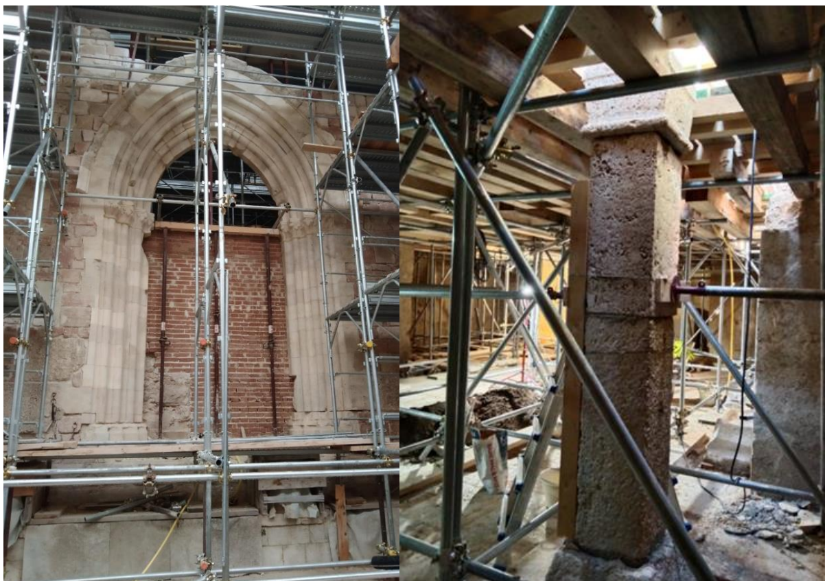
Left: The Gothic arch repositioned in the wall of the Basilica; right: one of the pillars repositioned in the crypt © MiC
