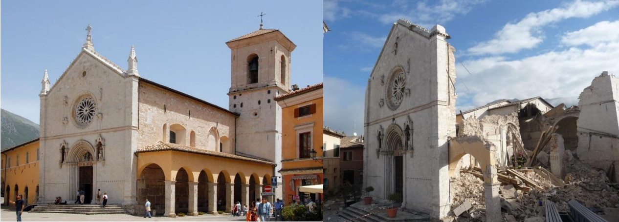
Left: The Basilica of San Benedetto in Norcia before and after the seism of 30 October 2016; right: the rubble masonry literally crumbled, leaving inside the Basilica a four meters high rubble front © MiC
