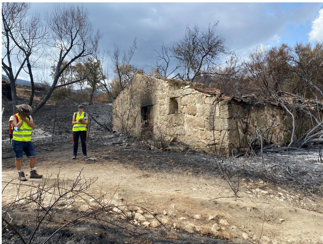
Field damage assessment © Terra Levis/UGRECYL
