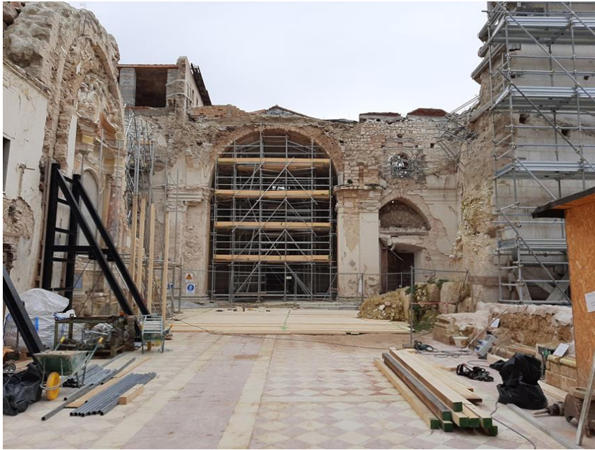
Basilica of San Benedetto in Norcia after the debris removal © MiC
