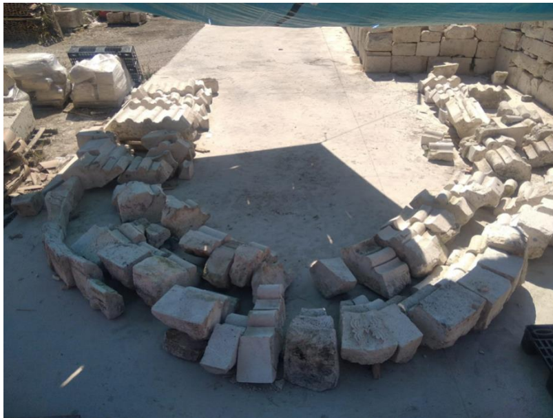
The Gothic arch reassembled at the St. Scholastica site with a view to its relocation © MiC
