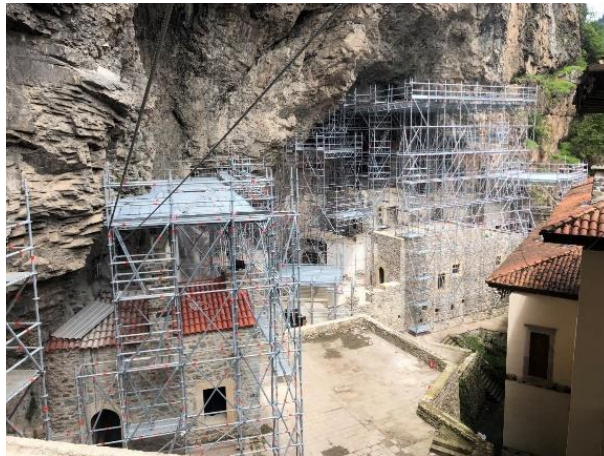
Courtyard scaffolding © MoCT
