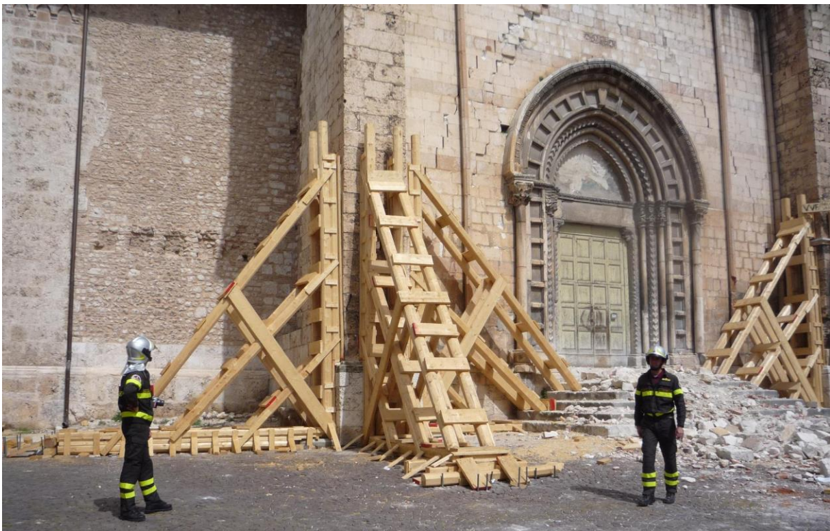
Fig. 4 Church of San Domenico (L'Aquila): Implemented provisional works © Vigili del Fuoco
