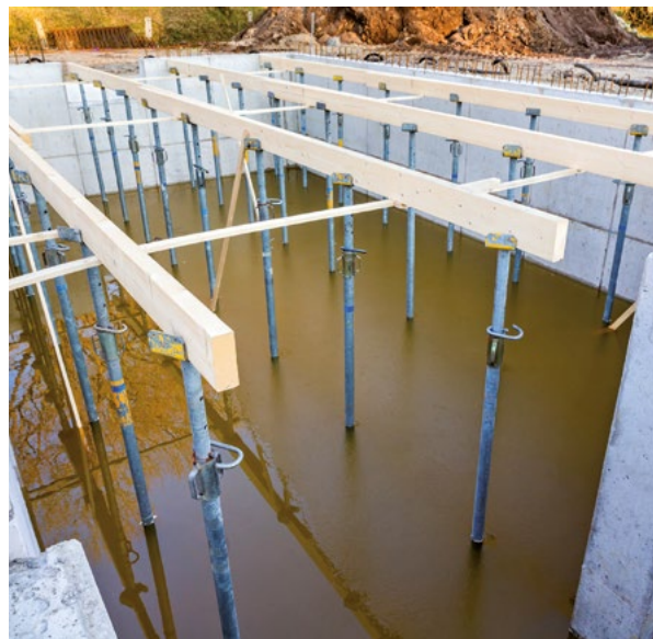
Now as before, there are still new settled areas developing in flood plains. (Photo: © benschonewille / stock.adobe.com)
