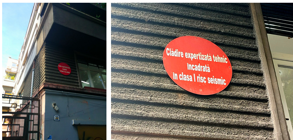
Figure 9 - A first seismic risk-class building in Bucharest marked with the red stamp.
