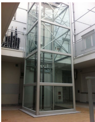
Figure 43. a) Elevator with independent structure; b) Elevator with reinforced concrete structure.
