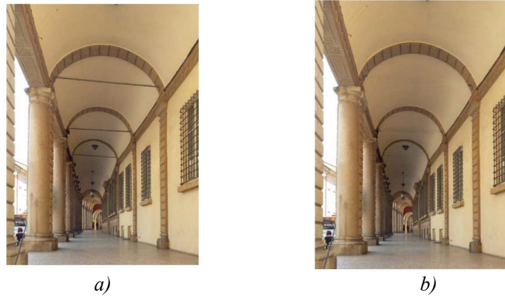
Figure 25. Type of barrel vaults a) with or b) without chains.
