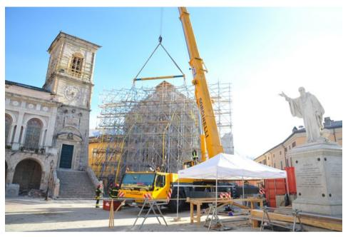
5. Installation of front steel tubes structure (Norcia, Italy 2016) © Corpo Nazionale Vigili del Fuoco
