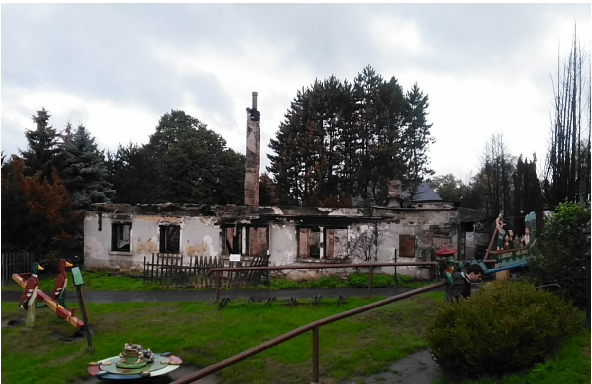
Figure 93. House destroyed by fire in the centre of Mezná. The house was not located close to the main burned area. The burning was likely caused by flying embers that ignited the coniferous garden hedges (right side).
