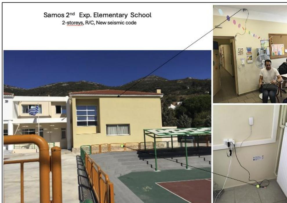
Figure 22. Vathy-Samos 2<sup>nd</sup> Exp. Elementary school building instrumented in ground floor and top ceiling.
