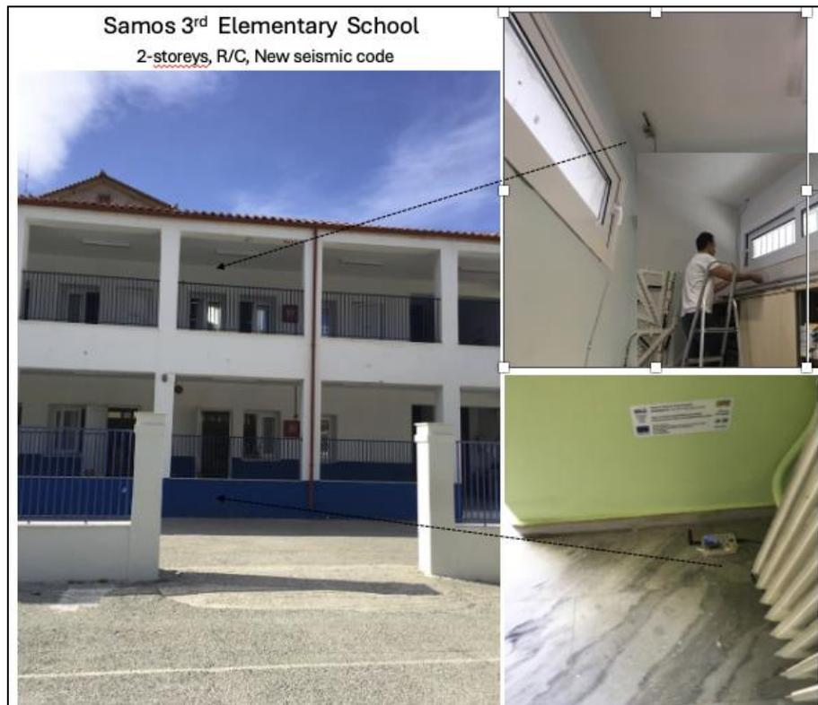
**Figure 23.** Vathy-Samos 3<sup>rd</sup> Elementary school building instrumented in ground floor and top ceiling.
