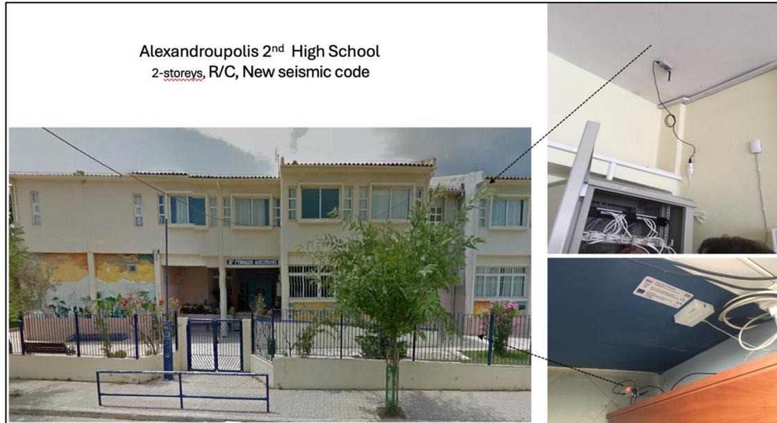
**Figure 17.** Alexandroupolis 2<sup>nd</sup> high school building instrumented in ground floor and top ceiling.
