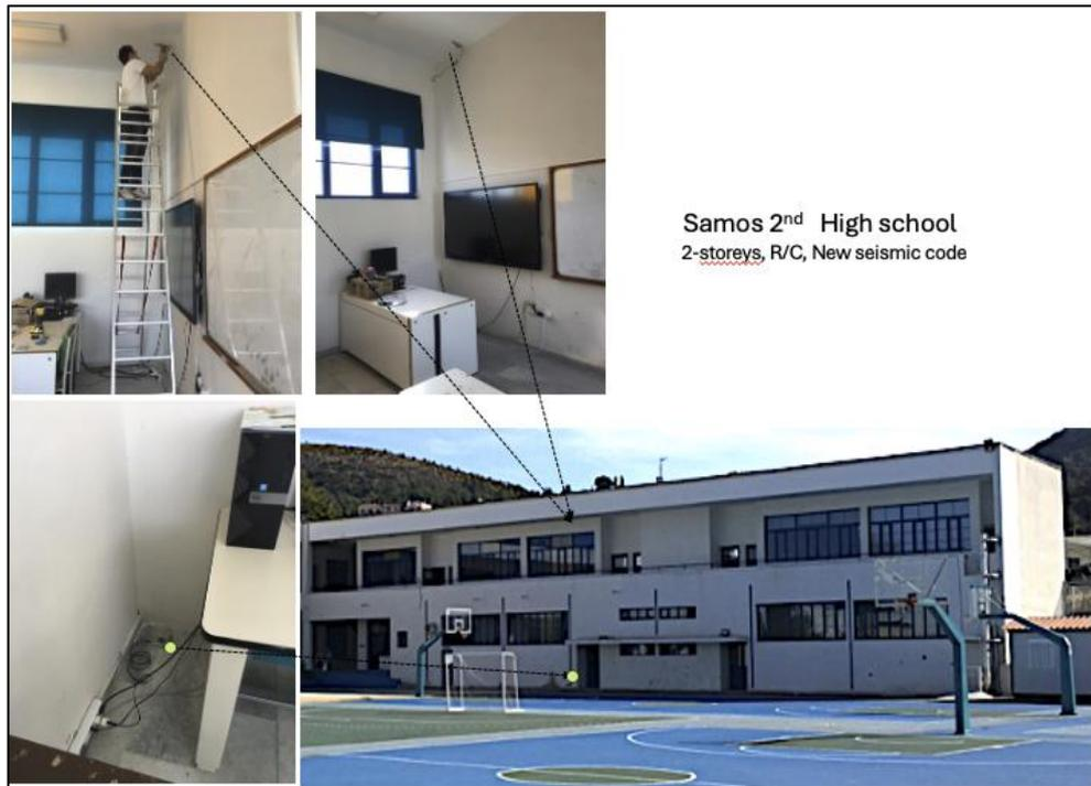
Figure 21. Vathy-Samos 2<sup>nd</sup> high school building instrumented in ground floor and top ceiling.
