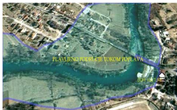
Figure 6.3: Flooded area during the December 2010 floods in Danilovgrad municipality (MPPFR Danilovgrad, 2014).
