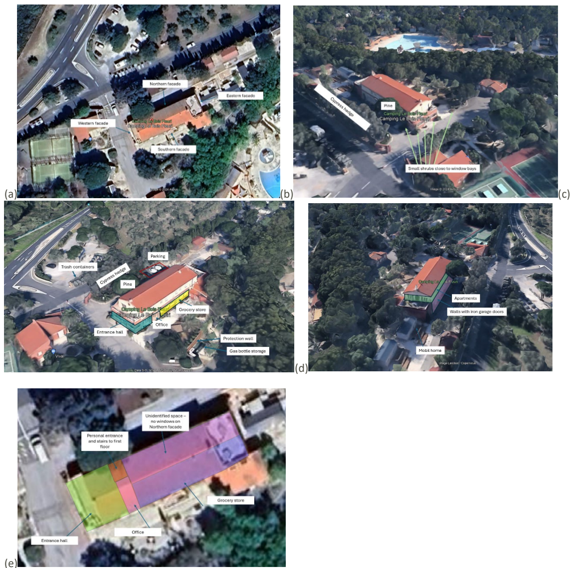
Figure 2-10 : Locations of other hazard and vulnerability items around entrance building: (a) view of facades, (b) view from Northern and Western facades, (c) view from Western and Southern facades, (d) view from Eastern and Northern facades, (e) ground floor basemap
