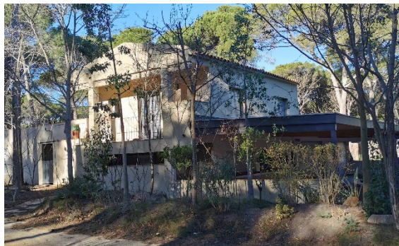
Figure 1: Left view of the building
