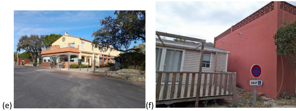
Figure 2-9 : Locations of different hazard and vulnerability items around entrance building: (a) unmanaged olive tree plantation on other roadside (historical photo before the 2023 fire), (b) cypress hedge at Northern façade being cut at 2m height, (c) large pine collocated to first stage of Northern façade, (d) isolated shrubs close to the window bay of entrance hall in Northern facade, (e) single small palm tree at Southern façade (among hardly flammable deciduous trees), (f) Mobile home close to Eastern facade
