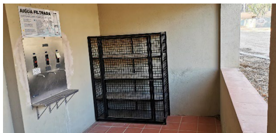
Figure 3: SCS with LPG canister storage rack
