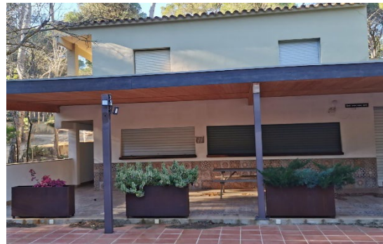
Figure 2: Front view of the building
