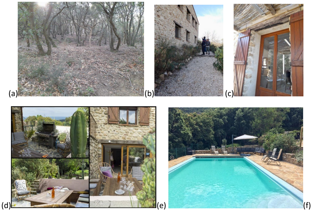
Figure 2-4 Locations of different hazard and vulnerability items around building: (a) cleaned surrounding cork oak forest, (b) Northern façade with ornamental vegetation, (c) pergola on Western façade, (d) and (e) garden furniture
