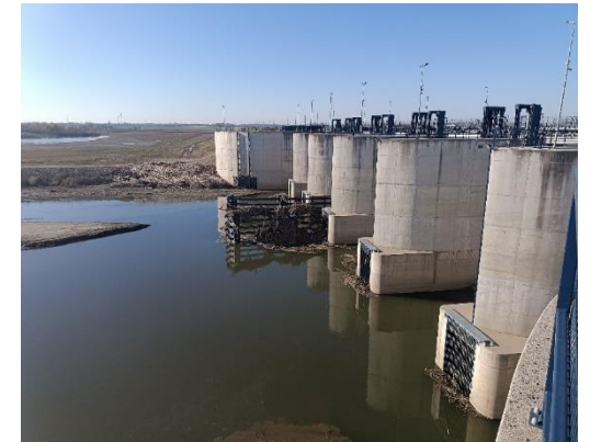
Racibórz Dolny flood protection reservoir
