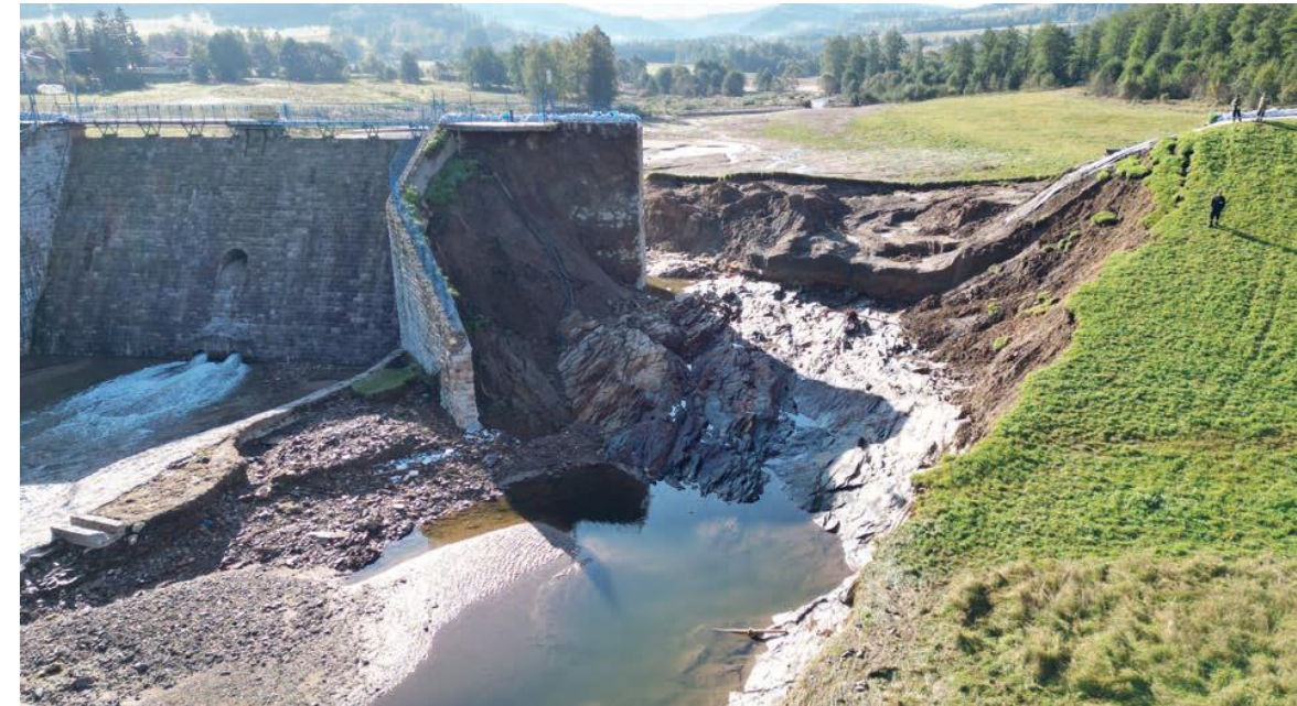
Stronie Śląskie. Broken dam on the flood control reservoir on the Morávka River burst. Photo S. Ostrowski
