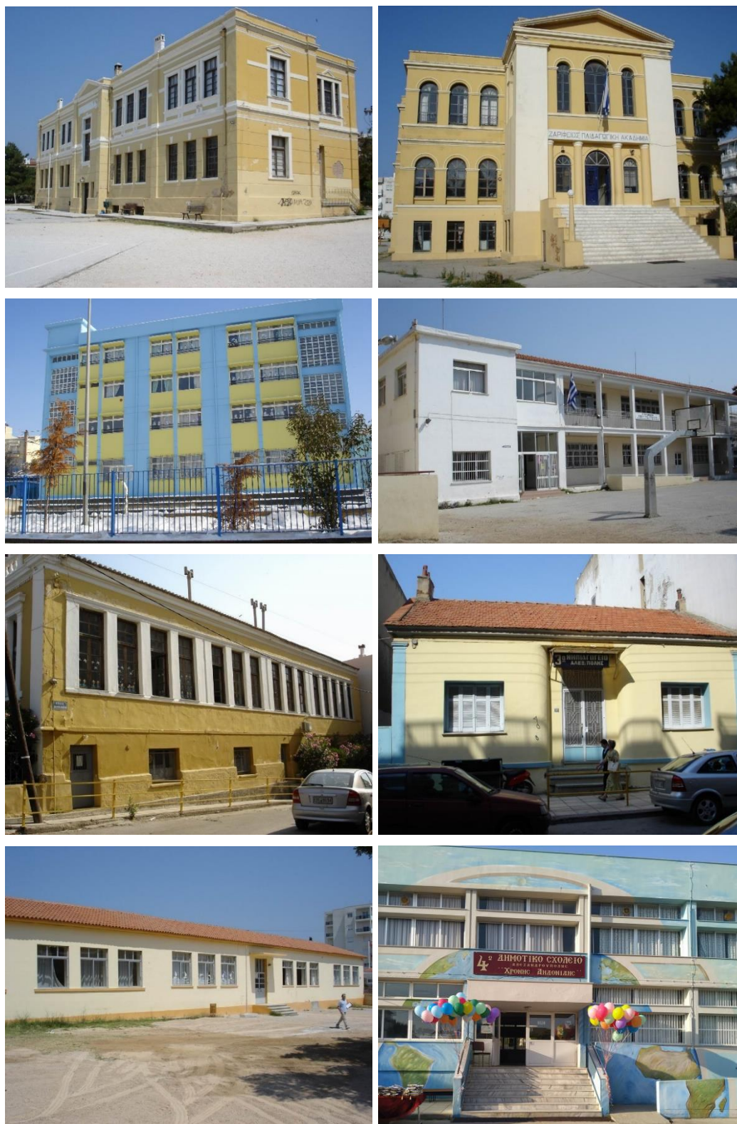
Figure 11. Various school building types in Alexandroupoli (mainly from the KT.YP. data)
