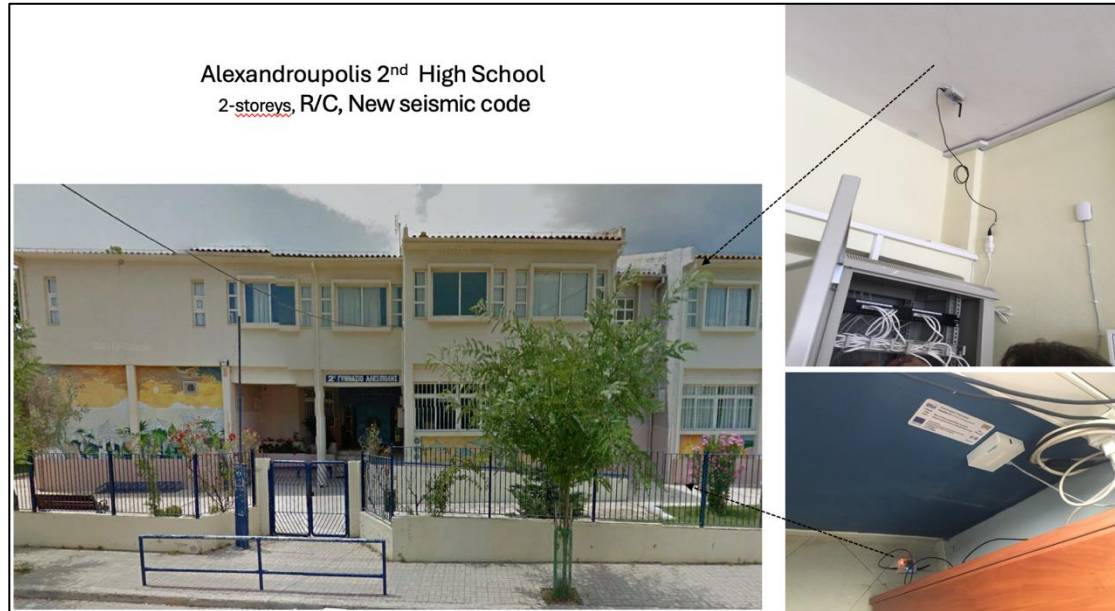
Figure 17. Alexandroupolis 2 nd high school building instrumented in ground floor and top ceiling.
