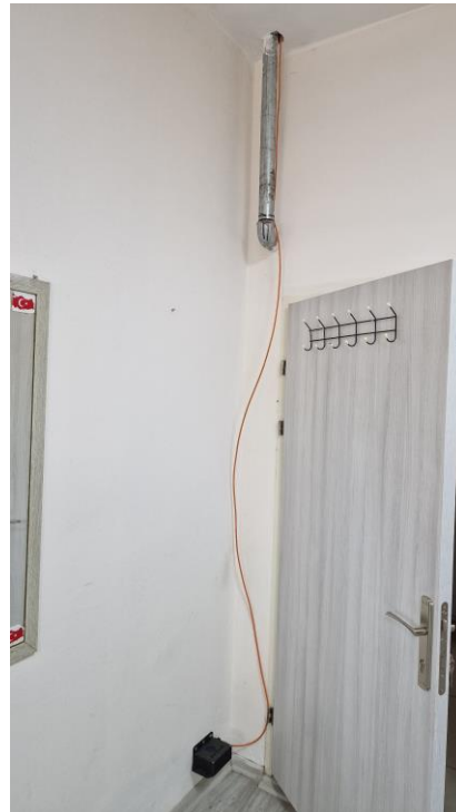
Figure 49. Çanakkale Anadolu Lisesi Basement Floor Accelerometer Location (Instrumentation).
