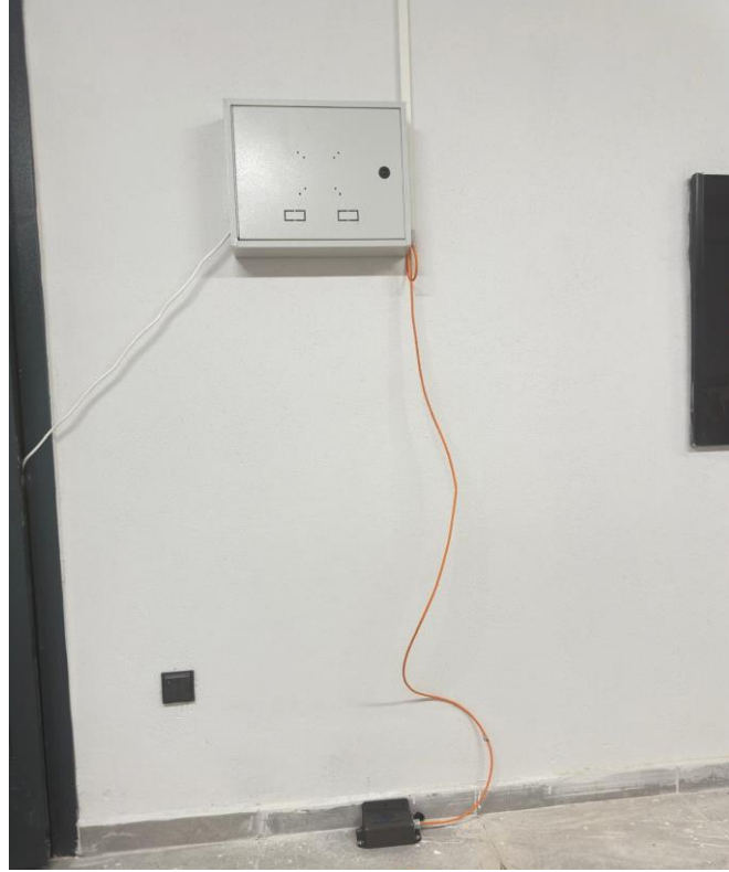
Figure 29. Çamkiran Ortaokulu Bayraklı 3 rd Floor Accelerometer Location (Instrumentation).
