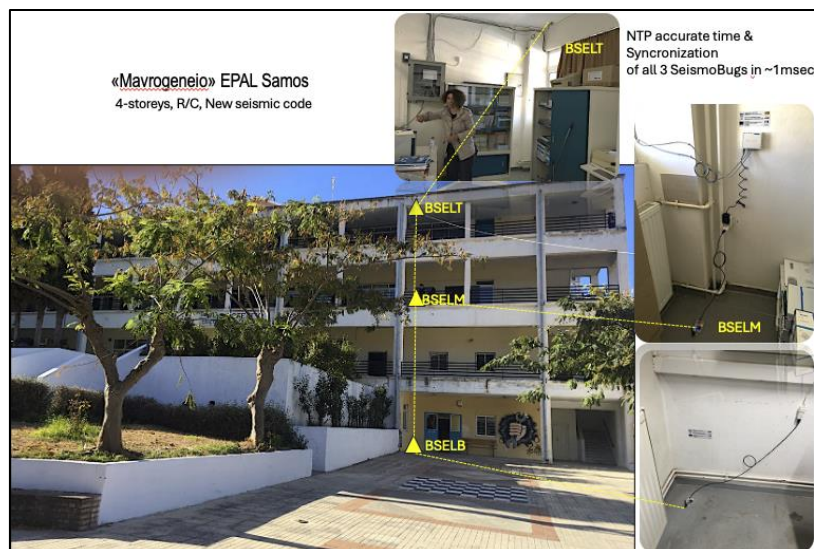
Figure 20. Vathy-Samos “Mavrogeneio“ EPAL building instrumented in ground floor, middle floor and top ceiling.
