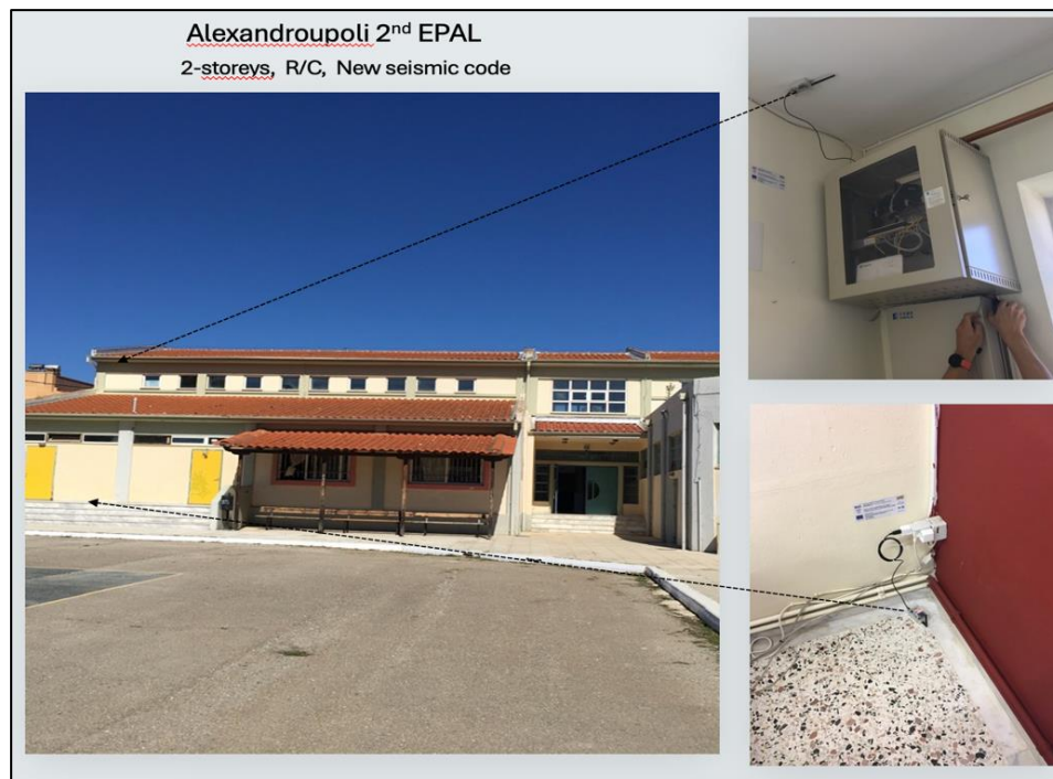
Figure 13. Alexandroupolis 2nd EPAL building instrumented in ground floor and top ceiling.
