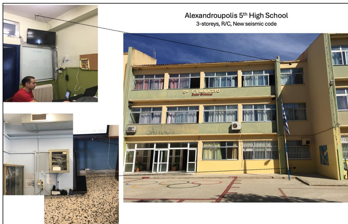
Figure 16. Alexandroupolis 5 th high school building instrumented in ground floor and top ceiling.
