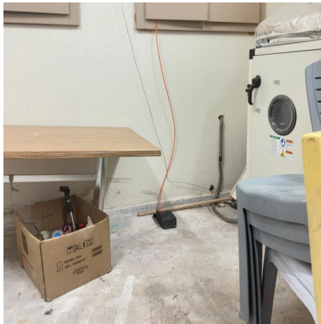
Figure 34. Buca Anadolu Lisesi Basement Floor Accelerometer Location (Instrumentation).
