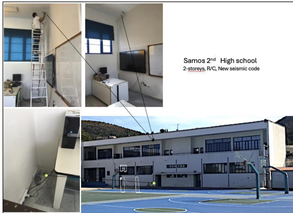
Figure 21. Vathy-Samos 2 nd high school building instrumented in ground floor and top ceiling.
