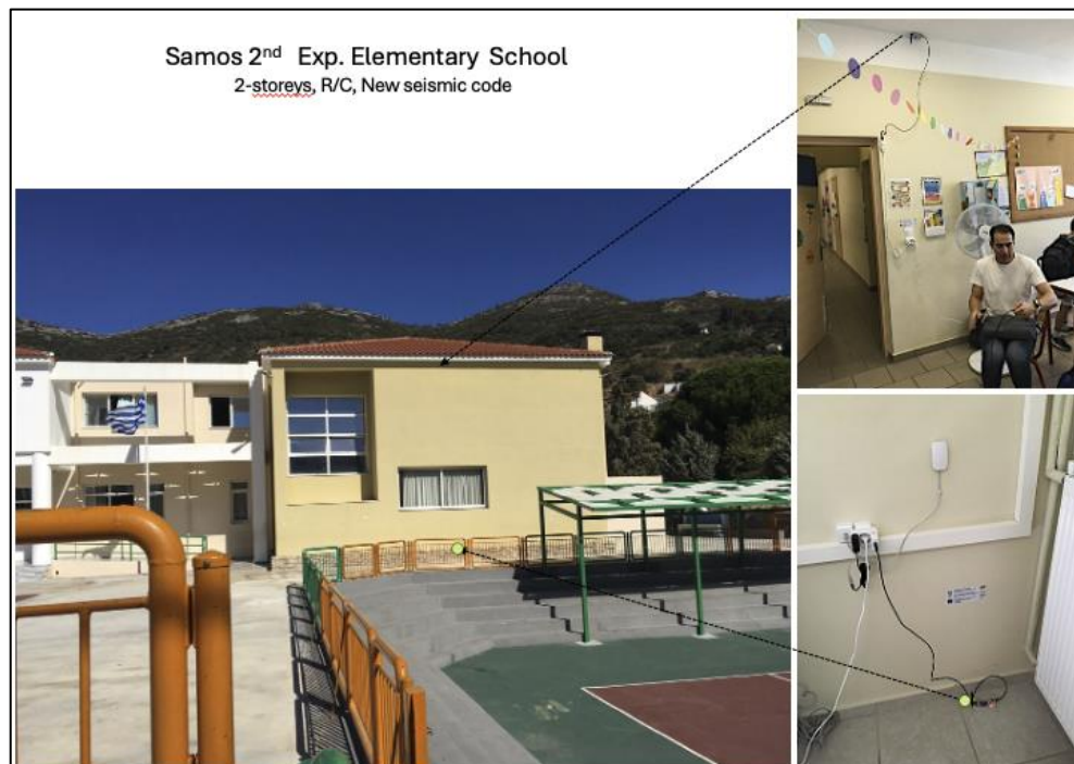
Figure 22. Vathy-Samos 2 nd Exp. Elementary school building instrumented in ground floor and top ceiling.
