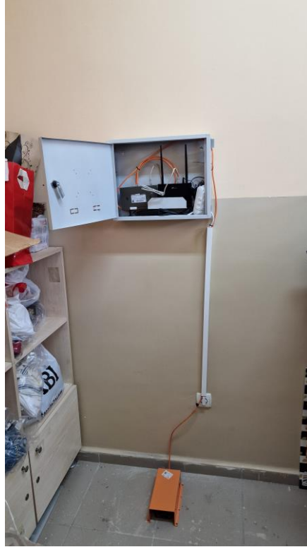
Figure 44. Cevatpaşa Ortaokulu 2 nd Floor Accelerometer Location (Instrumentation).
