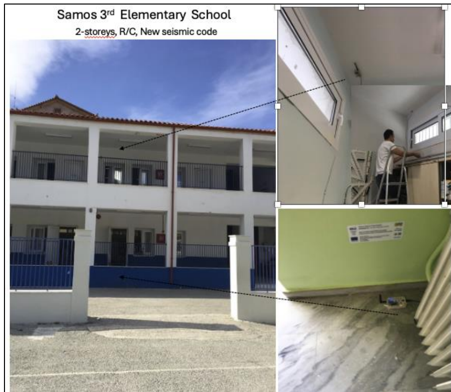
Figure 23. Vathy-Samos 3 rd Elementary school building instrumented in ground floor and top ceiling.
