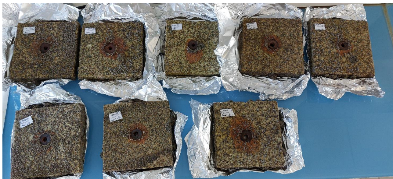
Figure 53 Pictures of the control tiles from the North face of the quay, after 11 months of exposure, at the laboratory before extraction
