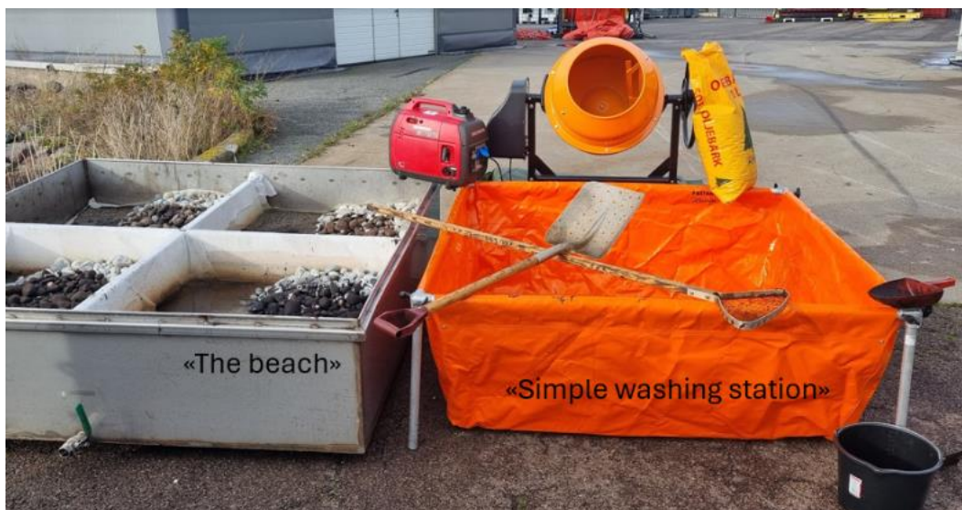
Figure 82: Simple version of in-situ washing station, without heated water or vacuum skimmer (if water temperature and tumbling is enough).
