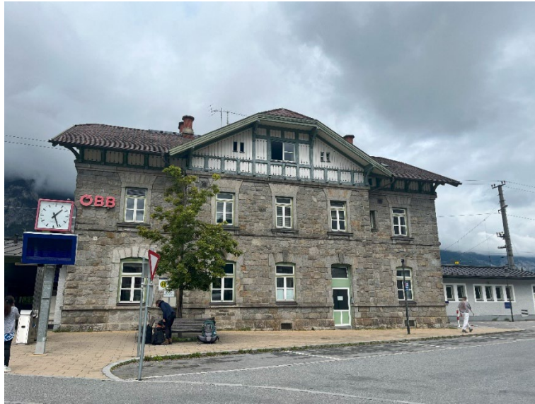
Figure 6. The railway connecting Austria to Switzerland is of European importance and goes through the municipality of Haiming. The train station (Ötztal Bahnhof) is a listed building.
