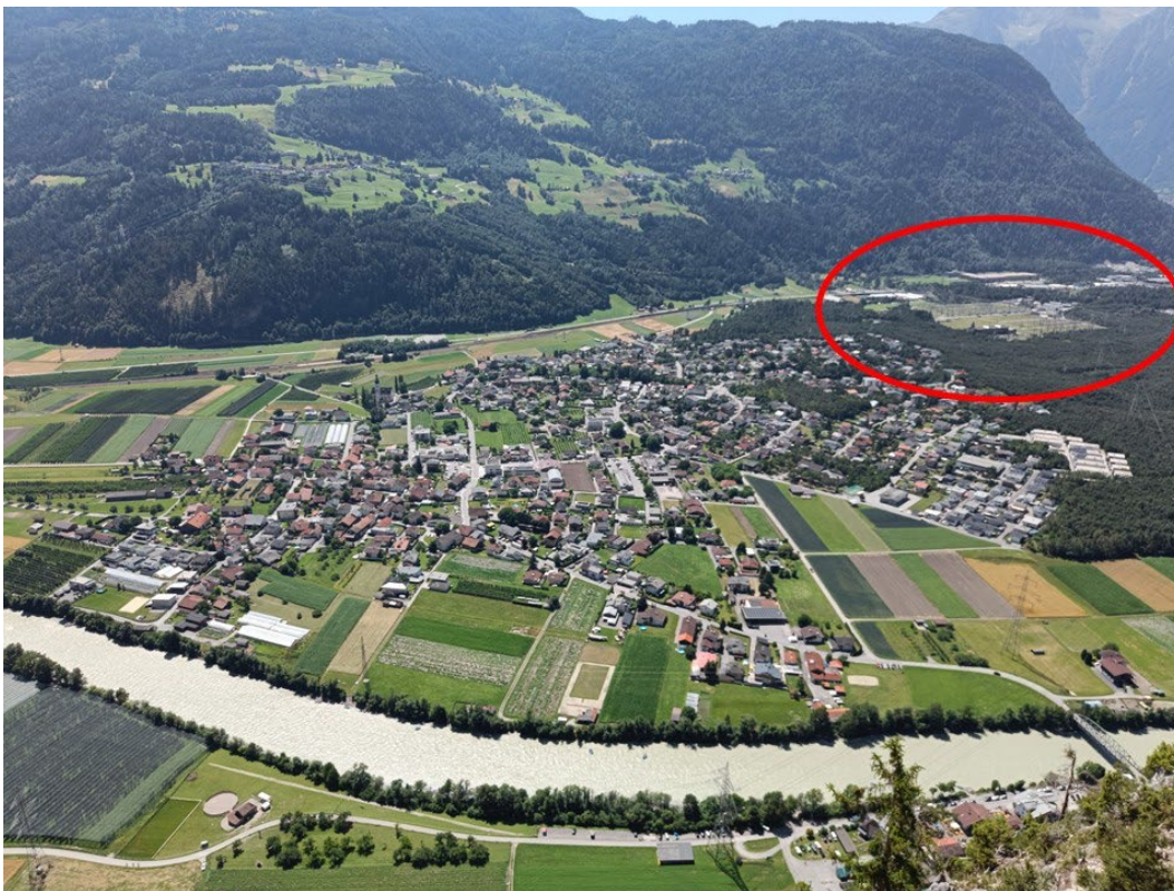
Figure 10. The location of the substation (red circle) in the municipality of Haiming (copyright Alfons Bauer CC-BY-SA4.0)
