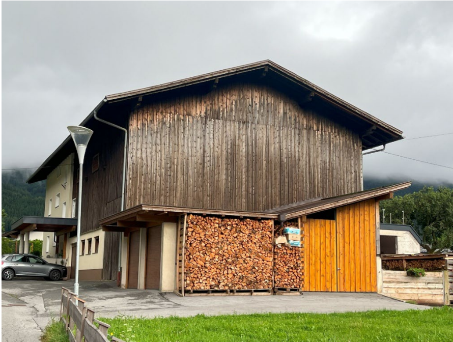
Figure 2. A typical Tyrolean building with adjacent wooden building for agricultural purposes and stored combustible materials.
