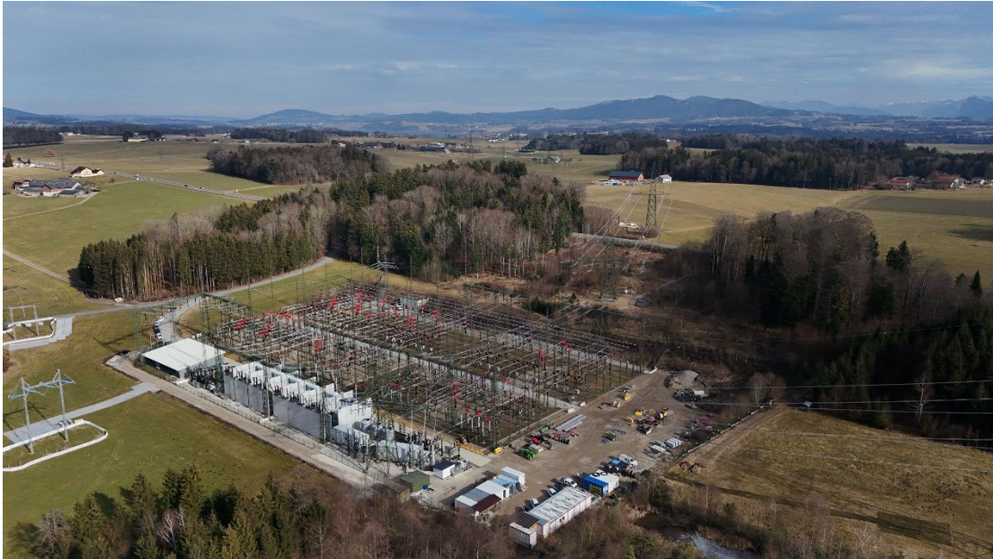
Figure 13. The electrical substation in Haiming. (Photo source: APG)
