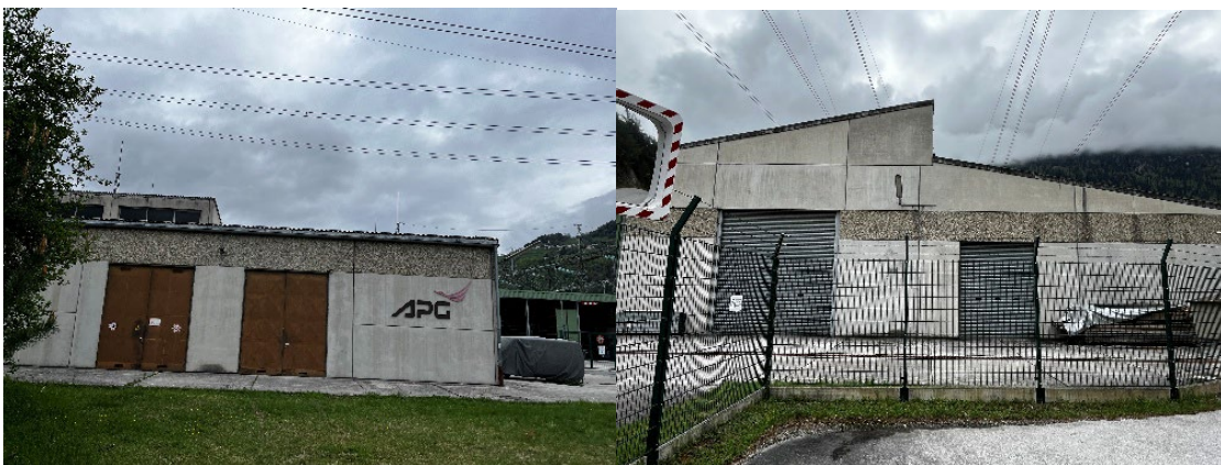
Figure 15. Buildings located within the territory of the electrical substation
