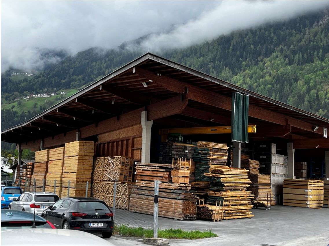
Figure 20. Industrial area in the WUI of Haiming in Tyrol, Austria (combustible products in the exterior of the building)
