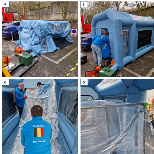
Figure 12. Inflatable primary and secondary enclosures for on-site VHP decontamination.
